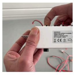
3 Push on the rear part of each LED spot in order to remove them from the gypsum block
